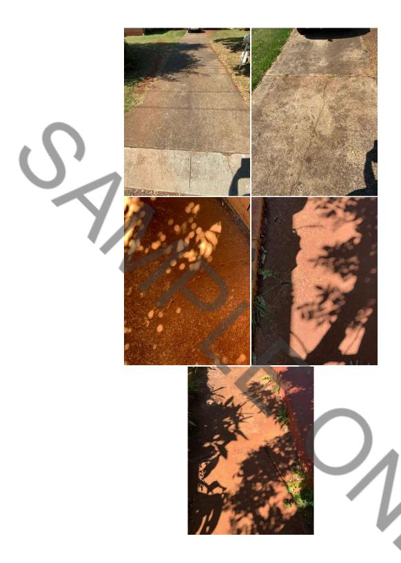
When cracking has occurred to the Pathways, these cracks are caused by product shrinkage during curing and/ or settlement. We are unable to determine the expected consequences on a visual inspection therefore you should consult a structural engineer to determine future consequences.
