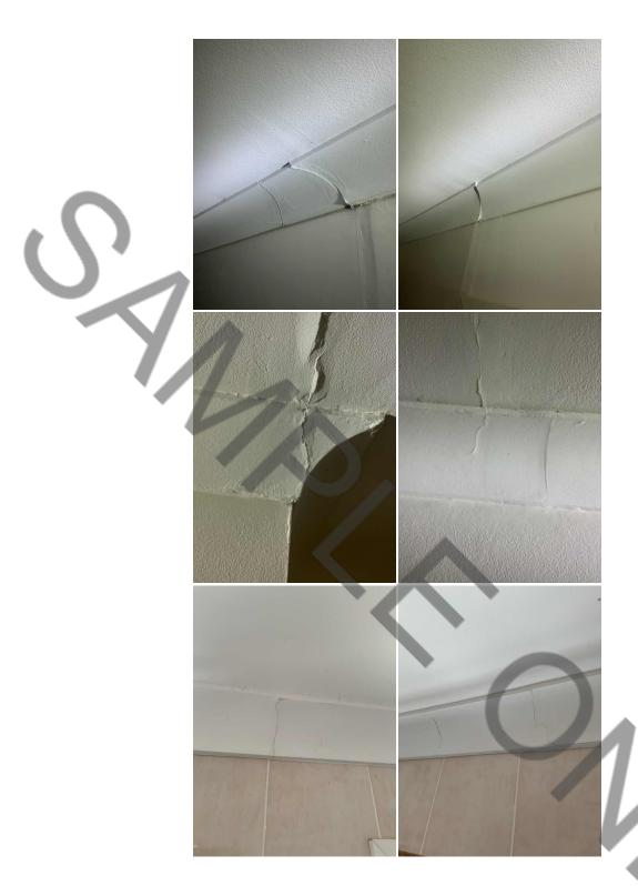
Minor cracking to the plaster/cornice are caused by minor building movement and settling and do not represent a long-term structural problem.
