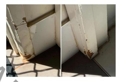
Defects should be referred builder for costing before you make your purchase. Timber rot or any termite damage will require a timber pest inspection and advice from a qualified pest inspector and also Builder for costing of repairs before you make your purchase, Invasive inspection is recommended to confirm extent of any damage.
