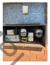
Earth leakage circuit breaker (Safety Switch) should be tested by a licensed electrician to determine if all power and lighting outlets are connected to this circuit and that it works. Meter box and switch boards require electrician to test and inspect, this is recommended before you purchase the property.
