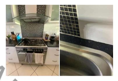
When the dwelling is furnished, heavily stored items including cupboards – restrict the inspector from a full inspection. No inspection under or behind kitchen cupboards. Joins at rear and sides of kitchen sink should be kept well sealed to prevent water penetration behind cabinet construction. You should consult a cabinet maker or builder before making your purchase.
